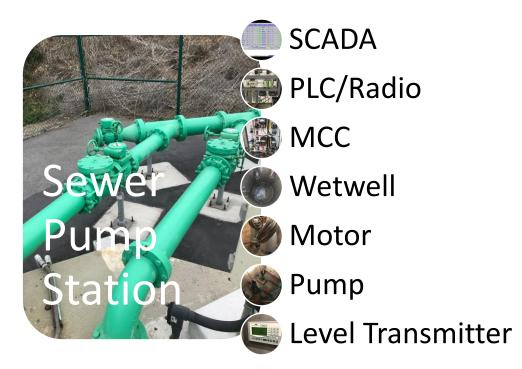
The District is comprised of 20 sewer lift stations that pump sewage from a lower elevation to a higher one, where it will then transition back to gravity. These lift stations are critical in keeping sewage flowing to the Monterey One Regional Wastewater Treatment Plant. The following Table 9 lists all the main assets of the District's sewer lift stations.
